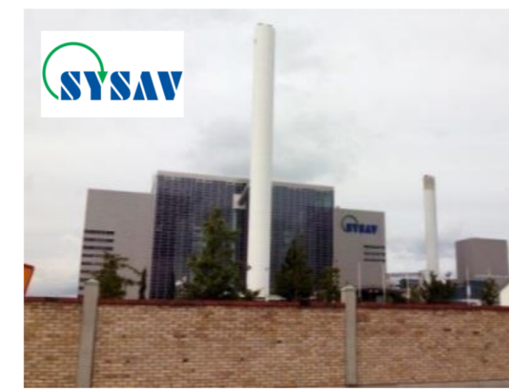
Sysav Waste management plant, Malmö, Sweden
